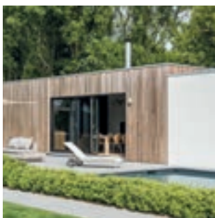
— timber framed buildings
